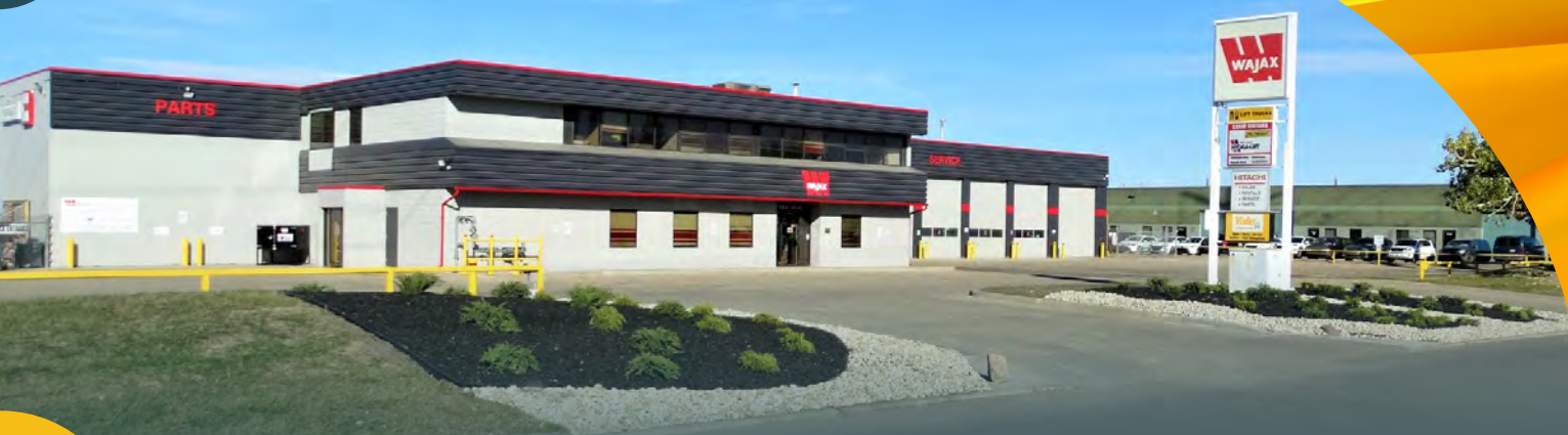
Wajax Building - Edmonton Acquired in 2020
