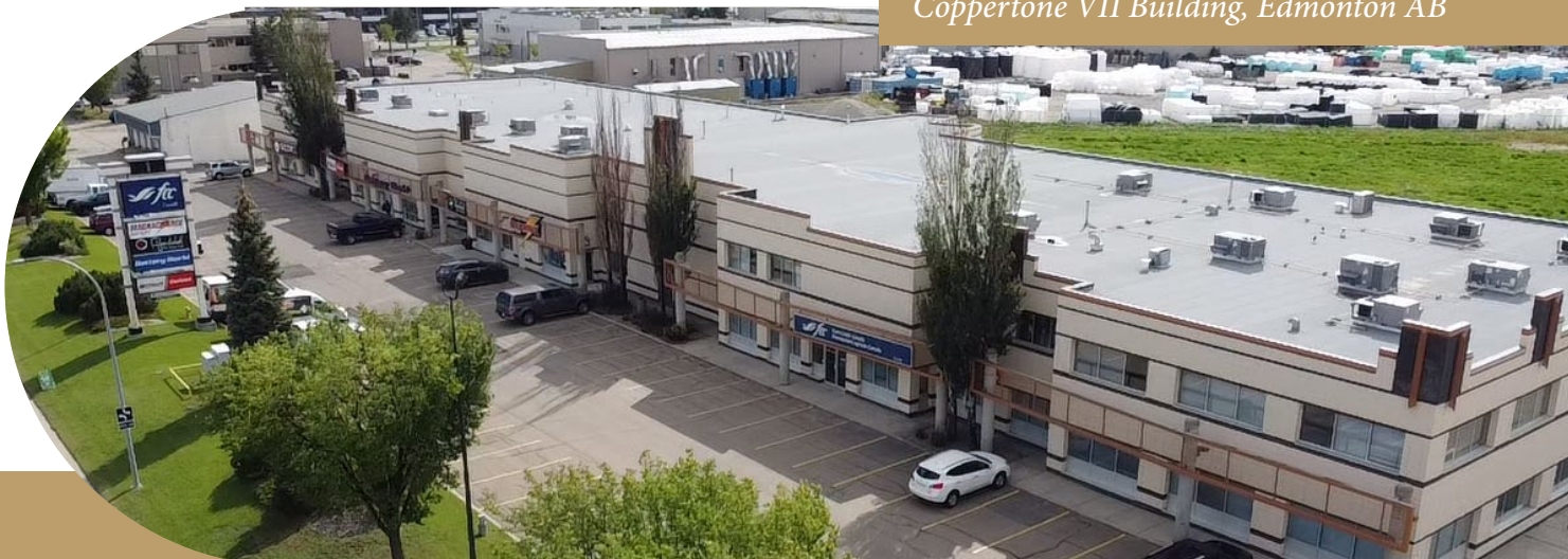
Coppertone VII Building, Edmonton AB
